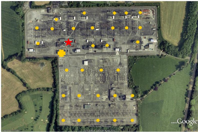
Figure 6 A WSN comprising free-standing radiometers insulation condition monitoring.
