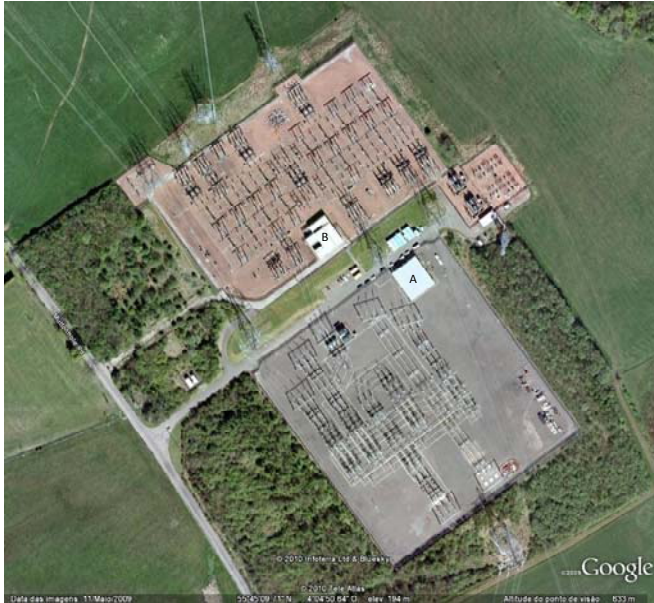
Figure 4: Location of measurement equipment (A) 400 kV control room, (B) 275 kV control room
